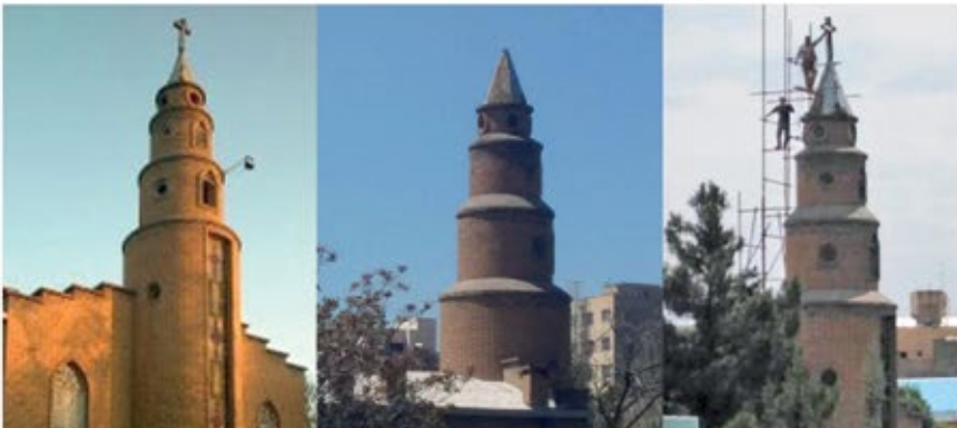
The Assyrian Evangelical Church in Tabriz with its cross, left, (viewed from the rear of the building) after the authorities tore it down on 9 May, centre, and with its cross restored on 9 July, right
